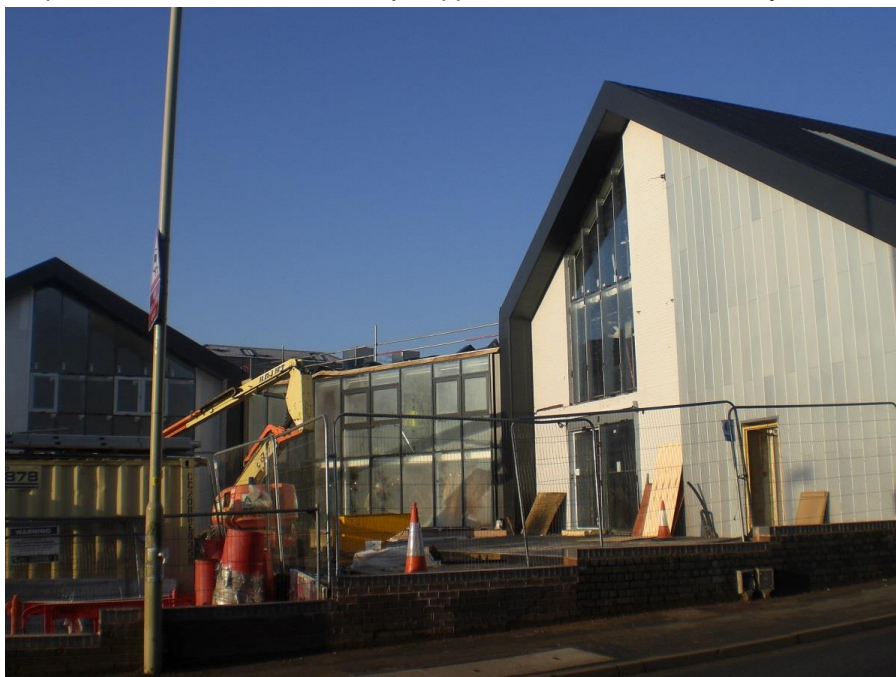
White House Cone Site 19.1.16
